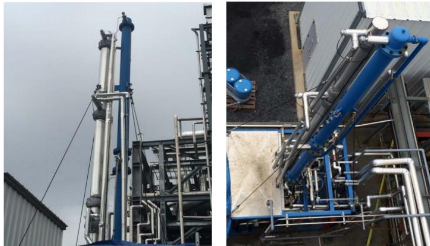
Figure 2: GPS-based skid used for bench-scale slipstream testing at NCCC
